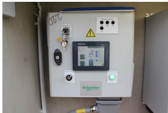
Control cabinet in separate ICT area of the compact station shown on the left
