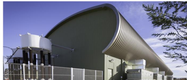
Converter Station Baixas 2 x 1000 MW (Source: Siemens)
