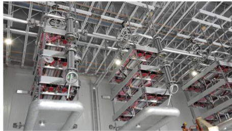
Installation von 500 kV Thyristor Valves (LTT) (Source: Siemens)
