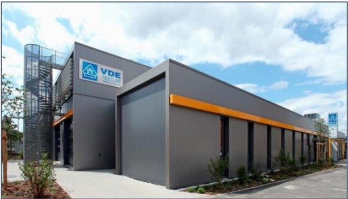
Figure 11. VDE’s BESS TestLab in Offenbach, Germany.
