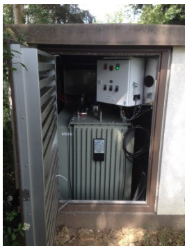
With the type of installation shown here, the transformer connections are safe to touch.
